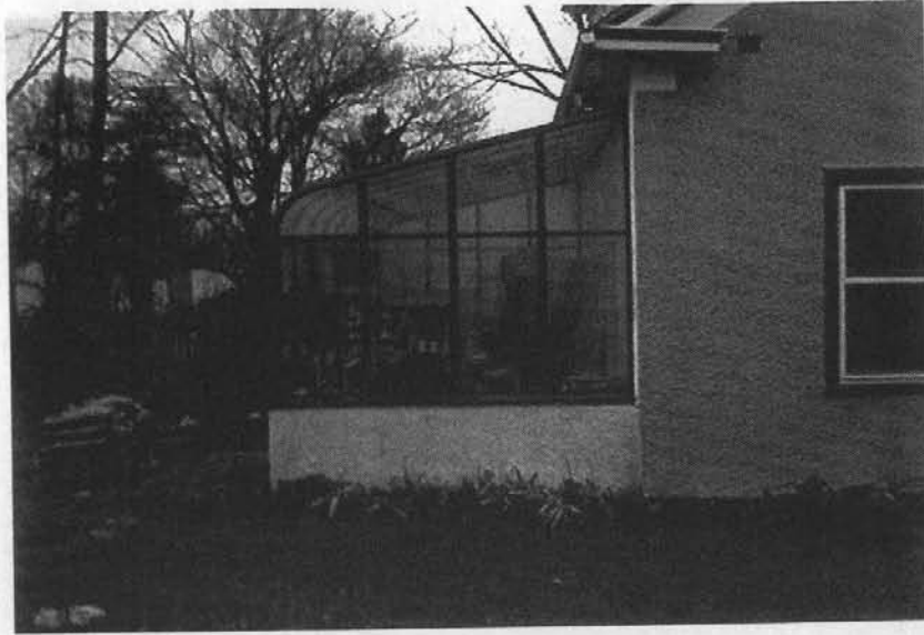
Existing Structure – Side View
