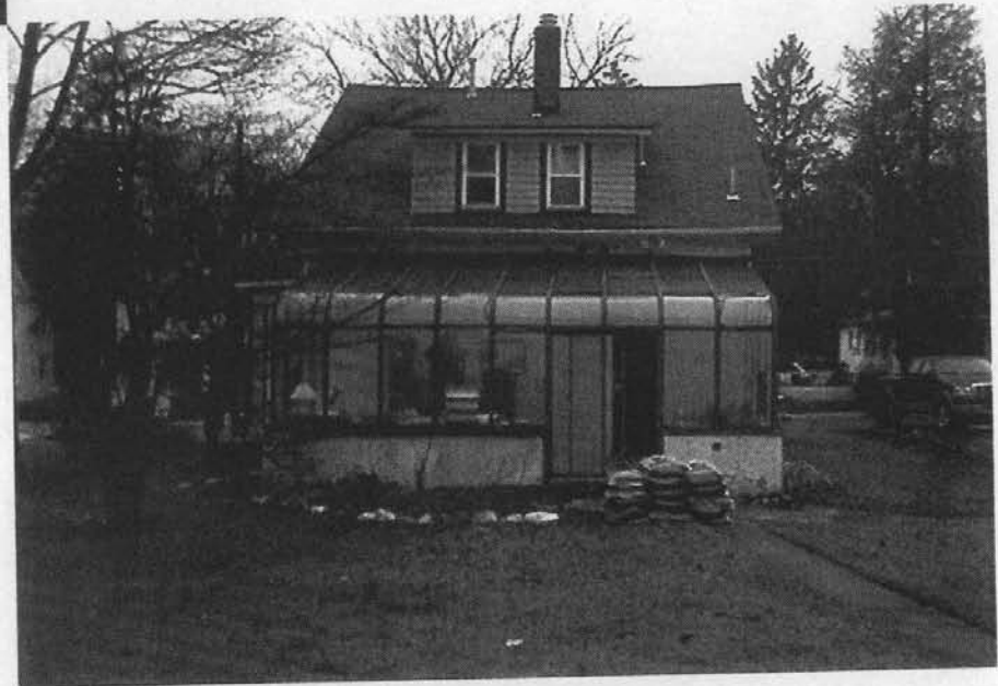
Existing Structure – Rear View
