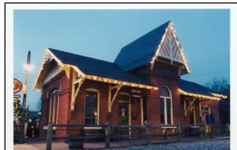
This historic train station in Olde Towne is still in use today on the MARC.
