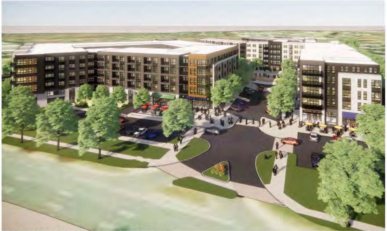
View C- Bird's Eye View Looking East From Frederick Avenue
