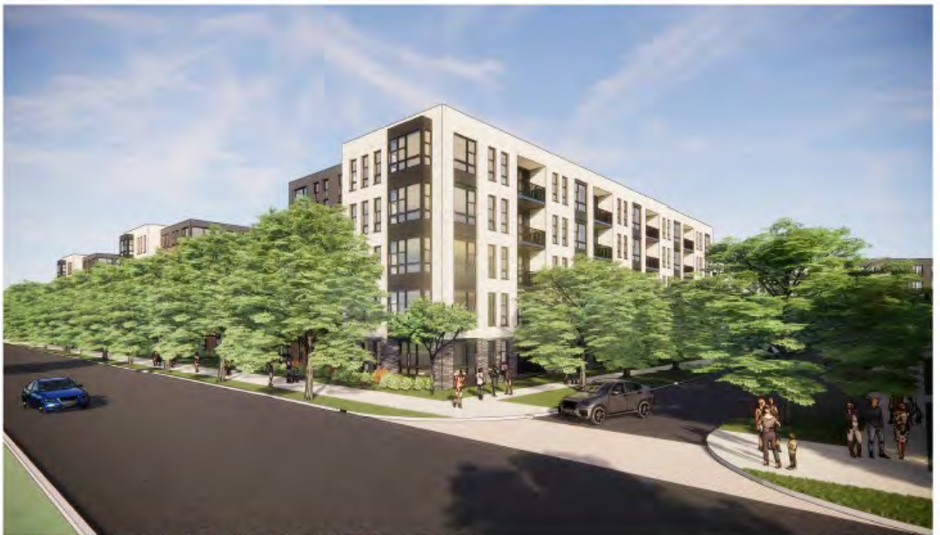
View D- Street View Along Travis Avenue
