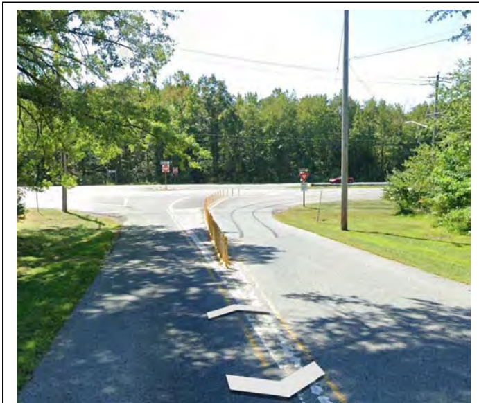
Flex Posts provide channelization to enforce right-turn only.
