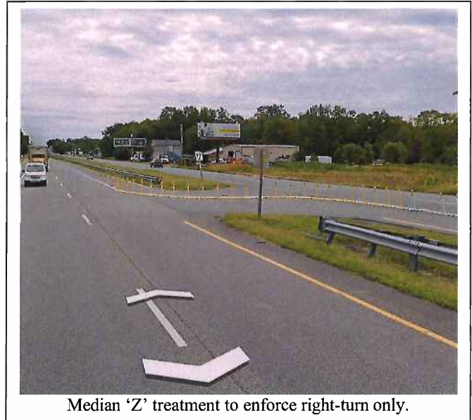
Flex Posts provide channelization to enforce right-turn only.
