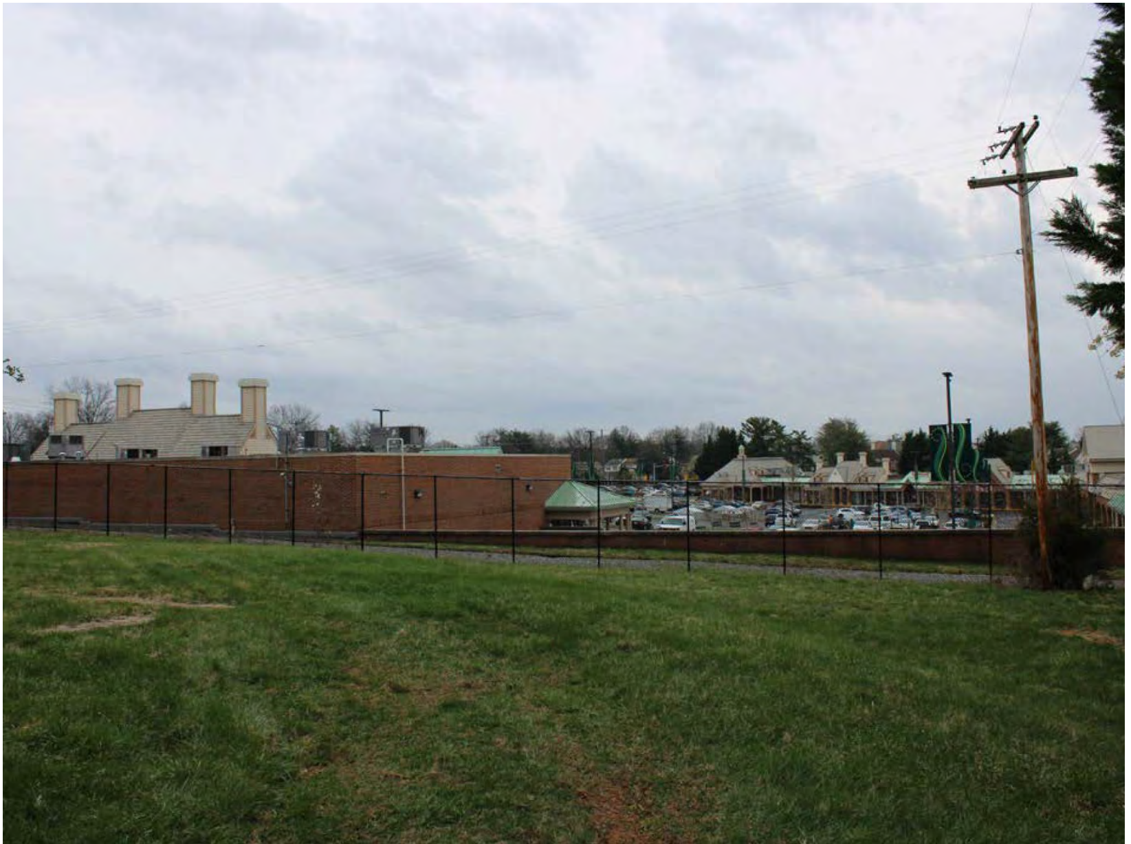
Adjacent Muddy Branch Square Shopping Center
