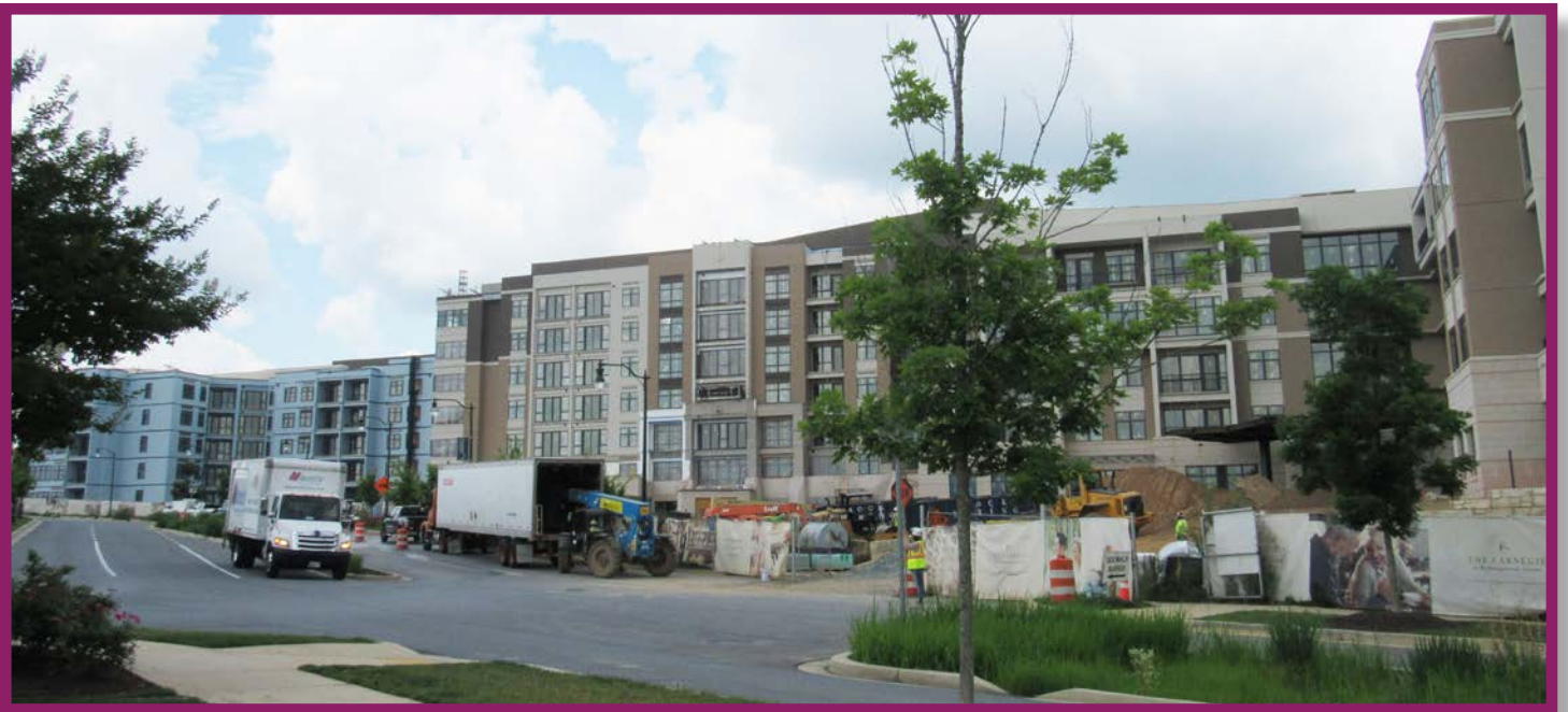
Construction of the Carnegie at Washingtonian Senior Residential Building
