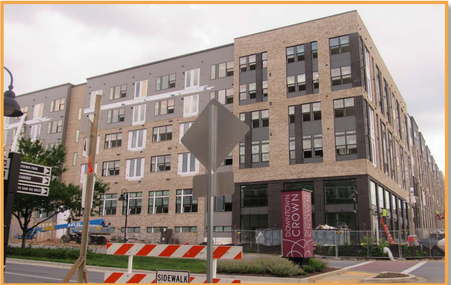
Multi-family Residential Building in Downtown Crown
