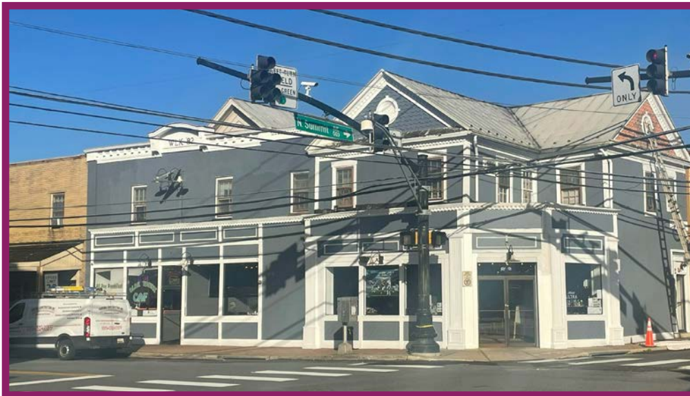
Exterior Improvements at 2226 East Diamond Avenue
