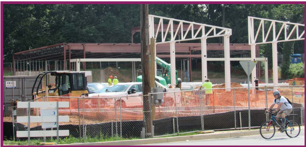
Wawa under construction on South Frederick Avenue
