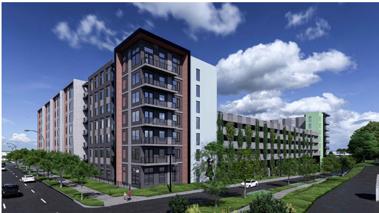
VIEW LOOKING NORTH - FROM N FREDERICK AVE
