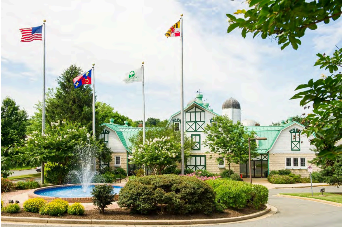
Casey Community Center
