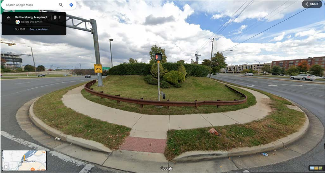
Existing Conditions 10009 Fields Road, Gaithersburg
