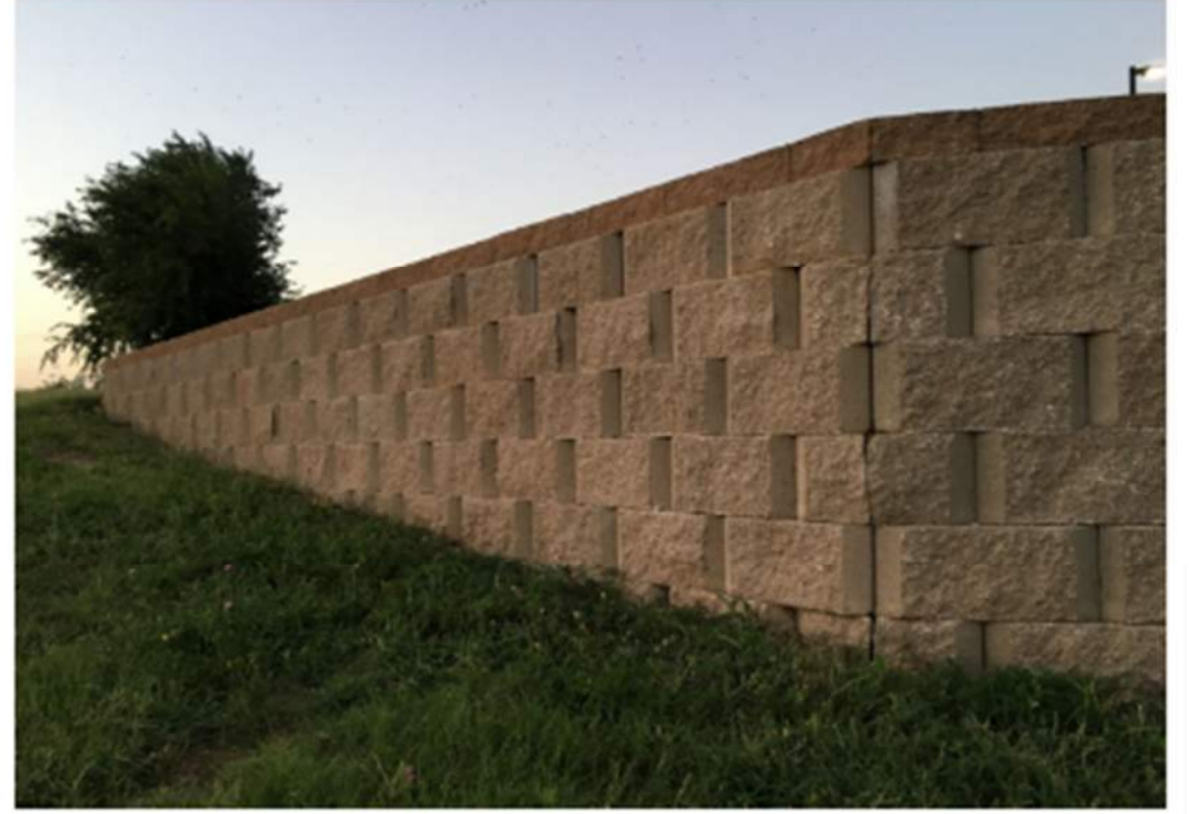
INTERLOCKING BLOCK RETAINING WALL EXAMPLE
