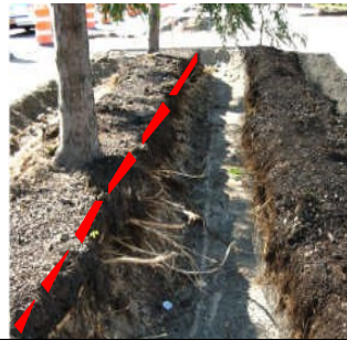
Figure 24: Note that for the example on the left only one pay line is needed as only one side of the trench requires pruning of live roots. The example on the right needs pay lines on both sides of the trench as there are live trees & roots remaining on both sides of the excavation.
