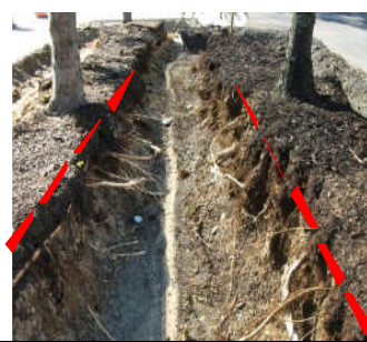
Figure 24: Note that for the example on the left only one pay line is needed as only one side of the trench requires pruning of live roots. The example on the right needs pay lines on both sides of the trench as there are live trees & roots remaining on both sides of the excavation.
