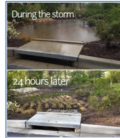
This bioretention garden drains water within 24-hours. Most will drain in two to three days
