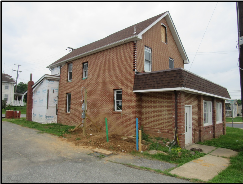
Exhibit 5. The north and east elevations of 102 South Frederick Avenue (June 2018).
