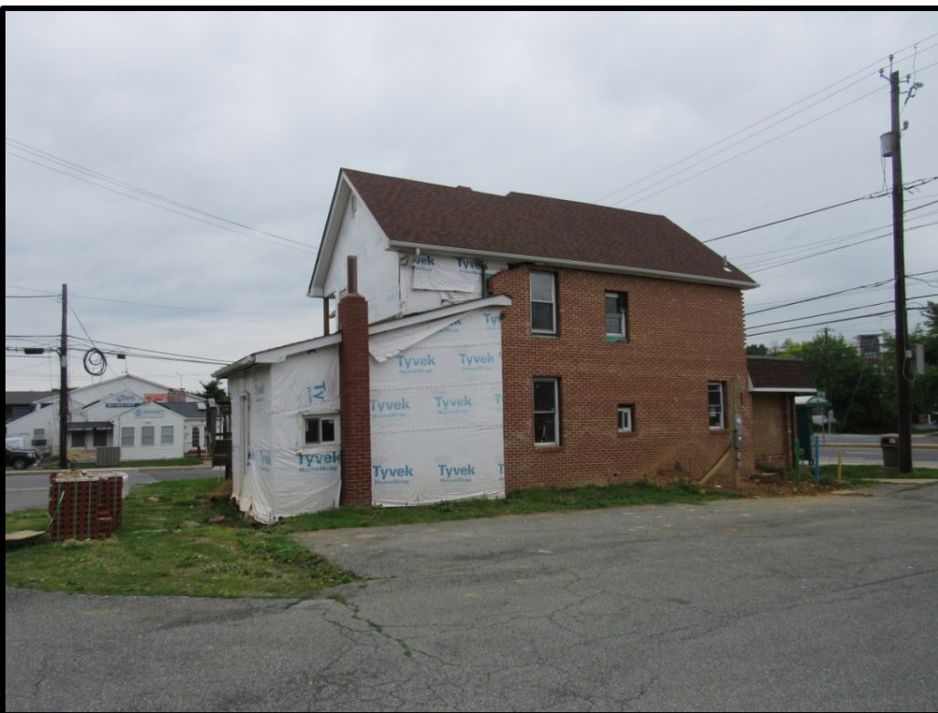
Exhibit 5. The east and south elevations of 102 South Frederick Avenue (June 2018).
