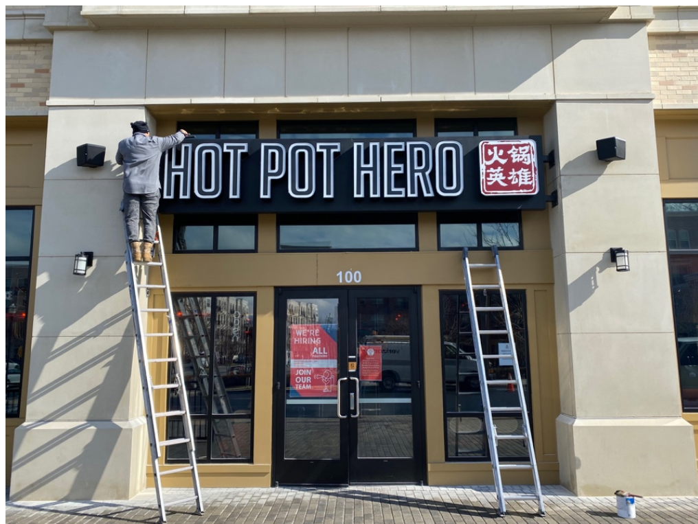
New Hot Pot Hero Sign suspended between precast columns
